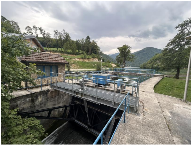
Segment Gate: stroke 1,5 m; width 6 m; high 3,4 m;
