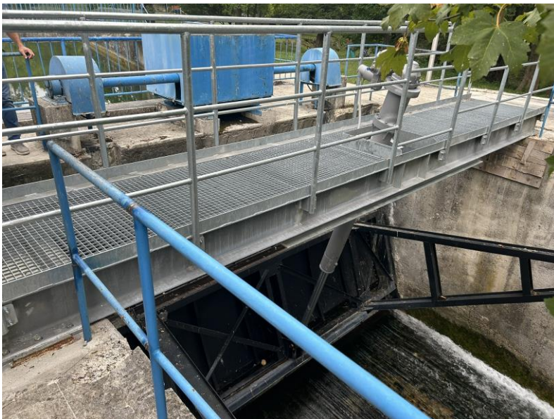
Electric Cylinder: Opening speed: 5 mm/s Opening time: 5 min for 1500 mm
